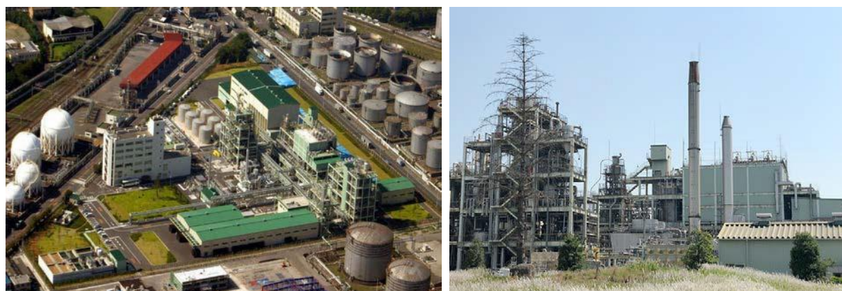
Figure 3-1 Appearance of the Plant
